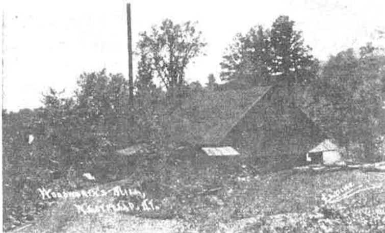
The Woodworth's Mill, Westfield, Vt., which was located just a little above Jean Meunier's house, 1913.
